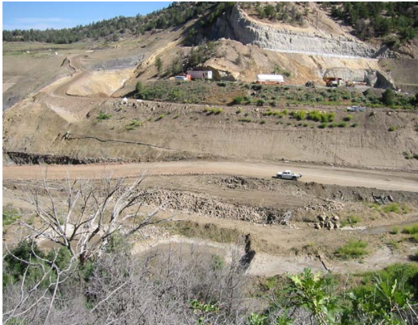
Construction activities at Basin Creek, view north.
