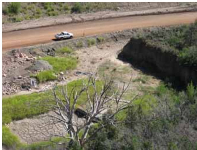
Construction activities at Basin Creek, view northeast.
